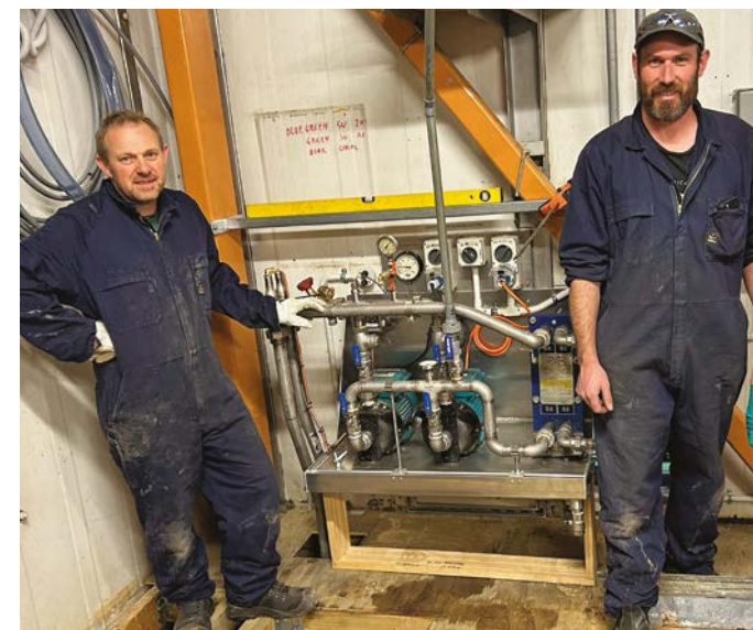
Upgrade completed to the glycol heating loop for the water intake. © Antarctica New Zealand
