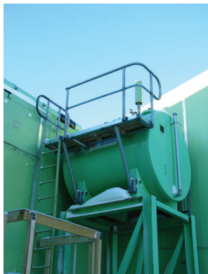
Figure 3b: 2,000 litre AN8 tank outside of the standby powerhouse.
