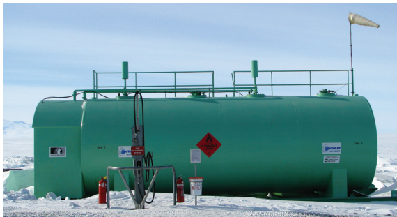
Figure 2: AN8 bulk tanks and vehicle bowser.
