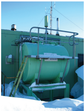
Figure 3a: 2,000 litre AN8 tank outside main plant room.
