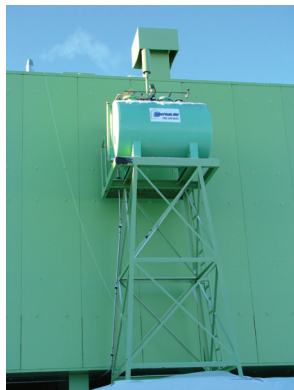
Figure 3c: 1,000 litre AN8 tank outside of HFC.
